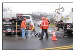
Place core cover on top of the Base, and open vents on top of core cover - ignite blower and position into baffle.
