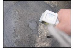
At 70° F ambient temperatures Utilibond will reach final strength gain in 30 minutes.
