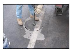
Remove the core heater and place the core in the opening, which will keep the core warm while mixing the Utilibond. Once ready, remove core, pour in mixed Utilibond, and reinstate the core as per normal procedure.
