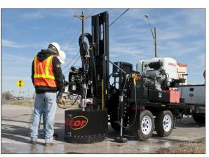
Left: Sam Inc. gets to work with MPX trailer mounted coring unit, making quick work of core cutting process through the roadway
